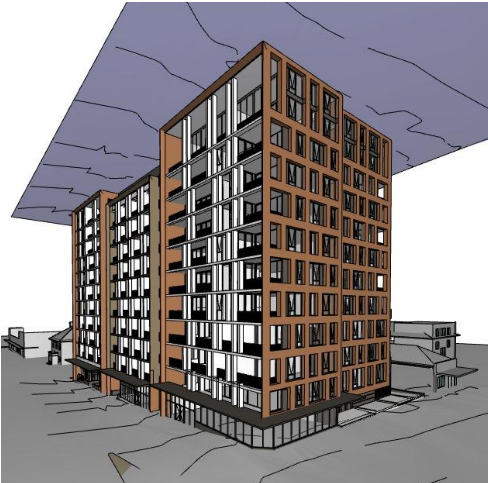
VIEW FROM MARY & PARK STREET INTERSECTION
